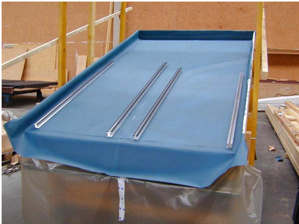
**Illustration 3: Element with Stamisol roofing-membrane**
