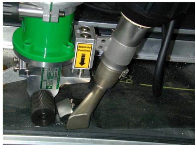
**Illustration 1: Welding of the element connection of the Novotan membrane**
